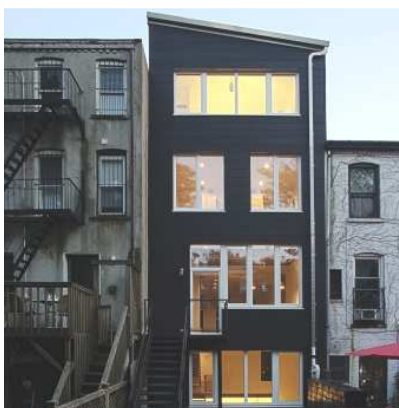
Tighthouse / Brooklyn (Sanierung in New York, USA). Foto: Hai Zhang
